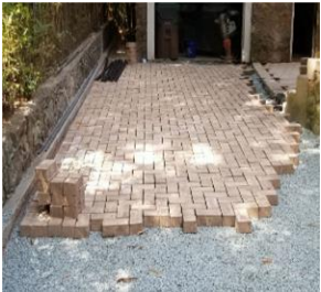
Driveway being constructed with pervious pavement
