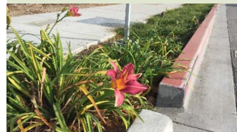
Bioretention area in the City of San Mateo
