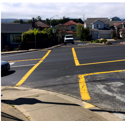
Figure 7. Crosswalk misaligned with the intersection corner at Chestnut Ave/Sunset Ave.
