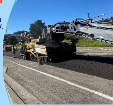
Downtown Area Enhancements: We're conducting critical concrete and asphalt pavement repairs to increase the longevity and resilience of our roads, preparing them for extensive sealing work ahead. In April 2024, the project will progress with important key tasks such as removing old striping, sealing cracks, applying surface sealant, and marking new lines. This will make our streets safer and more long-lasting.
